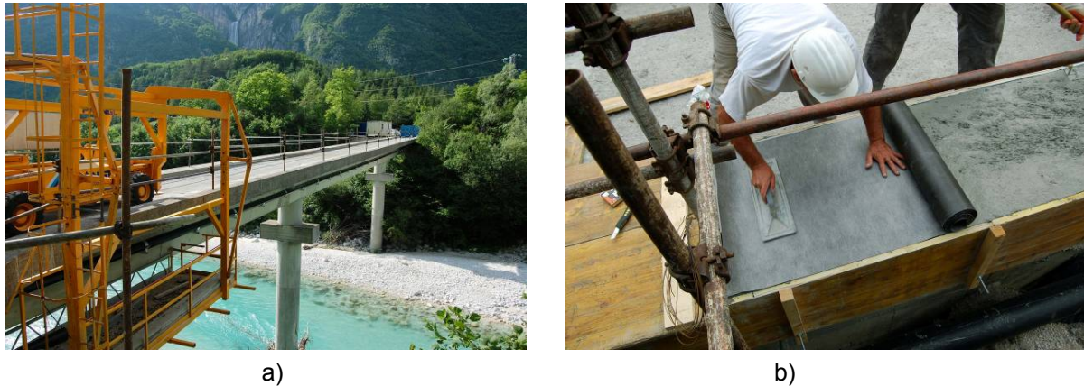
Fig. 2 a) bridge Log Čezsoški (nearby Bovec– Slovenia); b) Application of of a CPF membrane on the fresh UHPFRC of the footpath.
